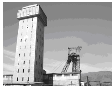
Fig. 4. Skip shaft winding engine
