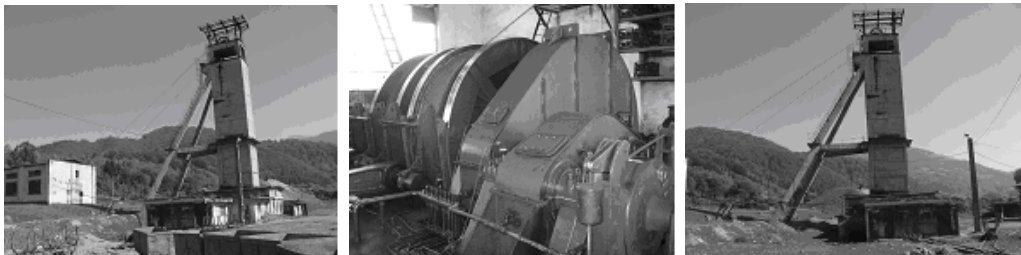
Fig. 1. Extracting installation Auxiliary well Jieţ “
